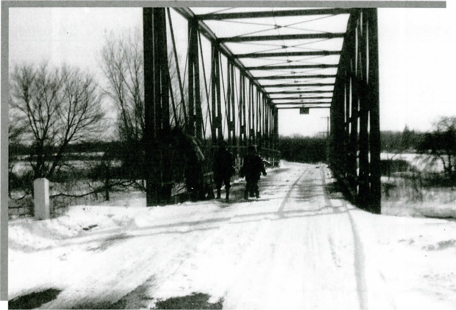
Old Iron Bridge, Meadville Rd., ca. 1940
