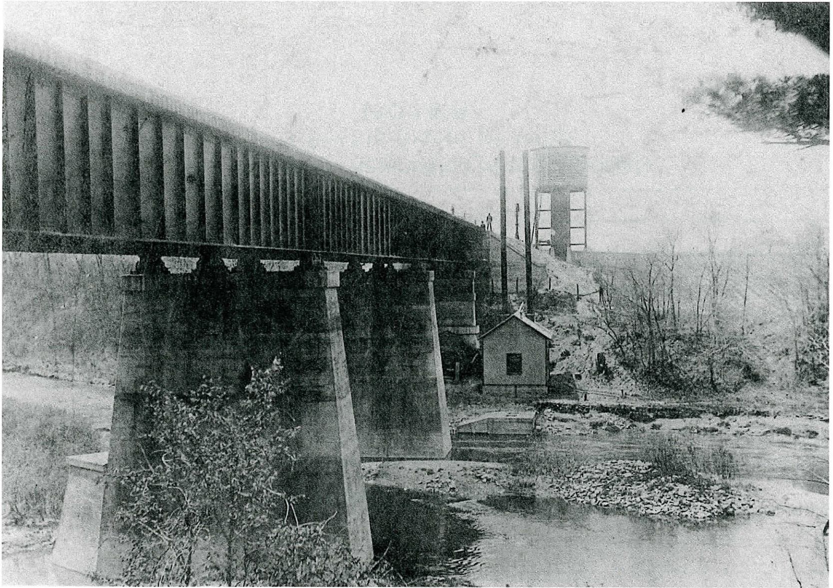
RAILROAD TRESTLE BRIDGE
